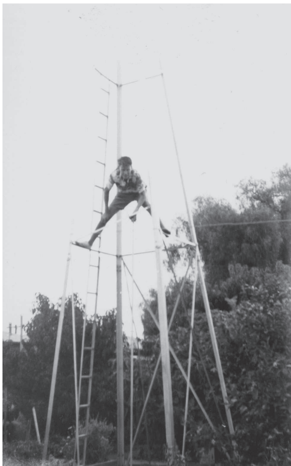
Doug McArthur perched precariously during assembly of his tower at Fullarton.
