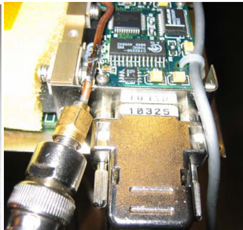
Left RF semi-rigid cable, right RS232 cable
